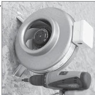
1. Mark the measure of **A** on the wall or roof and then fasten the fan.
